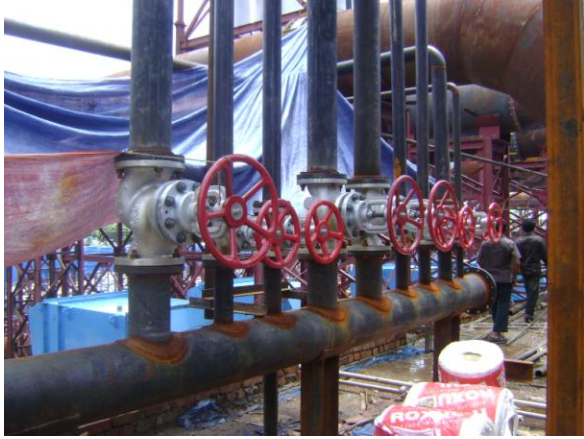
Steam Distribution Header and Versus Distribution Line at Gopalganj 108 MW (HFO) Power Plant.
