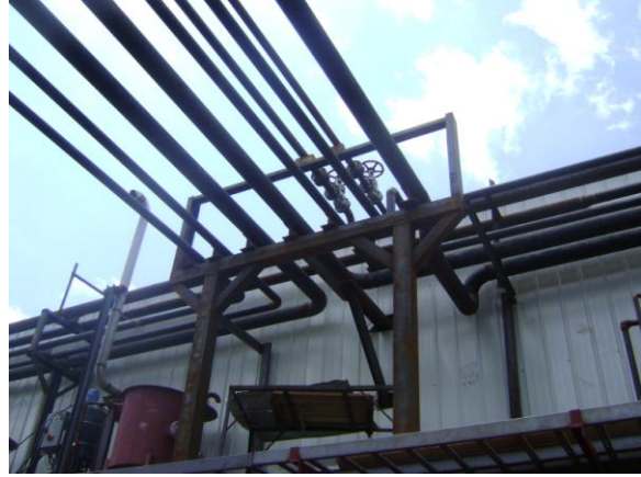
Steam Distribution Header and Versus Distribution Line at Gopalganj 108 MW (HFO) Power Plant.
